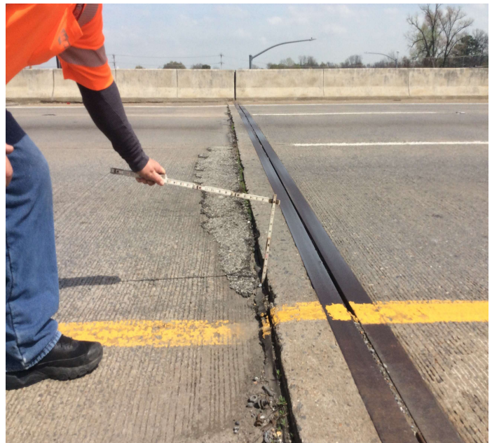
PHOTO 2 Description Eastbound north end of bridge inside lane has up to 2" settlement.
