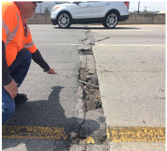
PHOTO 2 Description Bent 1 westbound, potholes in roadway at approach.
