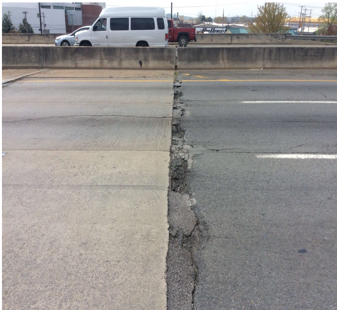
PHOTO 1 Description Eastbound north approach, large potholes.
