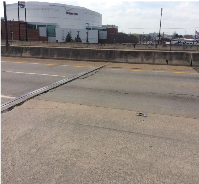
PHOTO 1 Description Eastbound north approach slab, large unsealed cracks and settlement on the outside lane.
