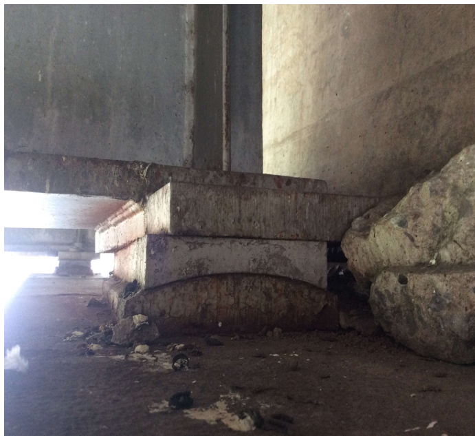
PHOTO 2 Description Bent 2 girder 2 bearing sliding out due to broken anchorage bolt.
