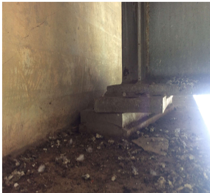
PHOTO 1 Description Bent 2 girder 14 bearing has slide half out.
