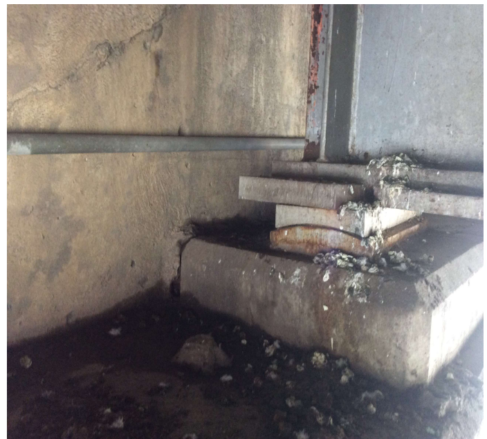
PHOTO 2 Description Bent 2 girder 10 is sliding out due to broken anchorage bolt.
