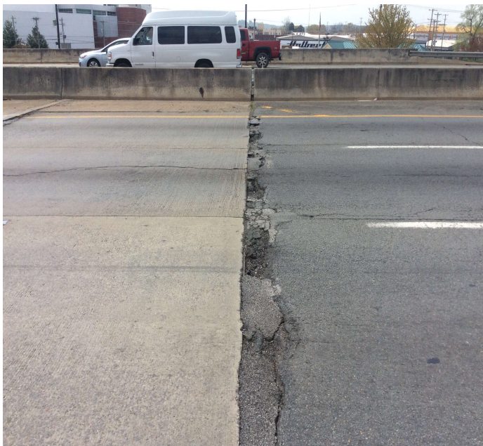
PHOTO 1 Description Eastbound north approach, large potholes.
