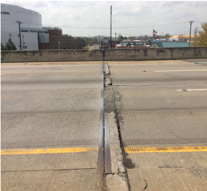
PHOTO 1 Description Bent 2 westbound large spalls filled with asphalt on top of back wall.
