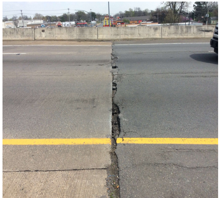
PHOTO 2 Description Eastbound south approach, potholes in roadway at the approach slab.
